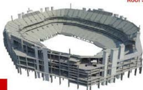
Main Concrete Structure
